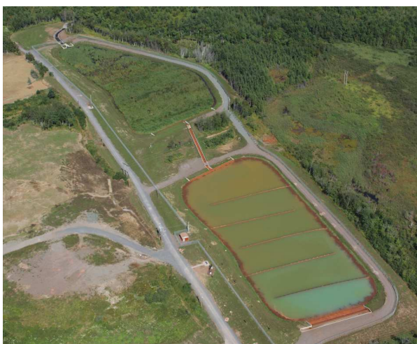
Fig. 2: An aerial view of the Neville Street passive treatment system (Cape Breton Island, Nova Scotia, Canada) with an aeration cascade at the bottom, followed by a settling basin and an aerobic constructed wetland at the top of the image (2010-08-29, © Langille Photos, Nova Scotia, for PWGSC and ECBC).
